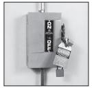
When preparing to remove or install a motor, put safety first. Wear appropriate personal protective equipment (PPE). Follow applicable electrical codes for wiring, disconnect and emergency stop requirements. Lock out and tag out all potential energy sources before working on the motor. Use safe lifting methods appropriate to the motor's size and weight.
